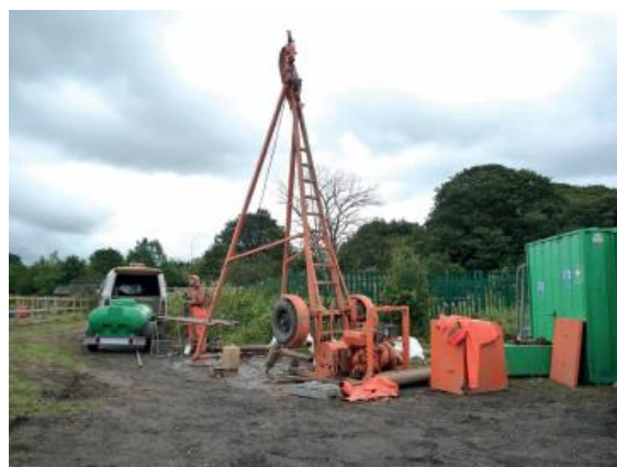
Cable Percussive Rig
